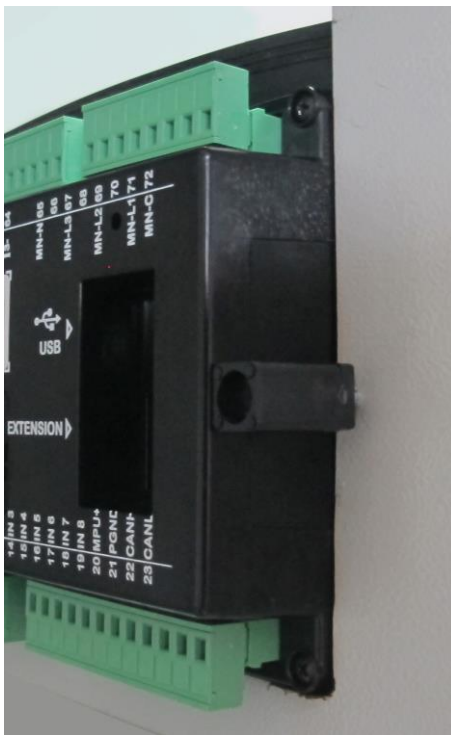
Installation of screw type bracket
